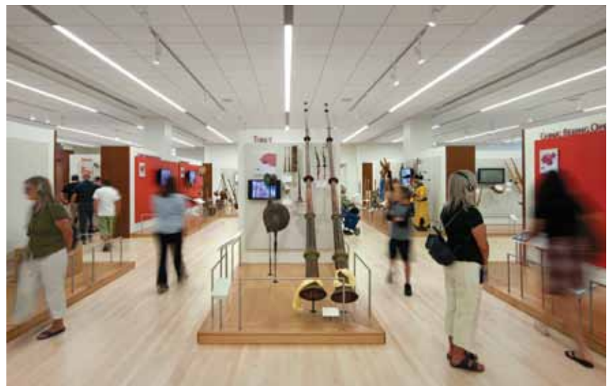
An integrated ceiling system at Phoenix’s Musical Instrument Museum, designed by RSP Architects, uses large, monolithic panels to coordinate all utilities and devices in the ceiling into a six-inch utility strip at eight inches on center.
